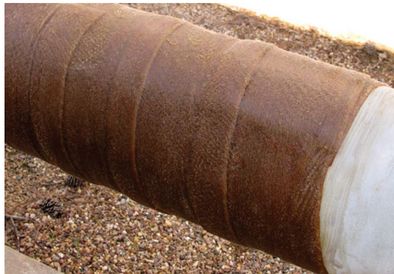
After coating with primer, the wrap should be wrapped onto the pipe in a spiral pattern using a minimum 1" overlap. Seams and ends should be sealed.
